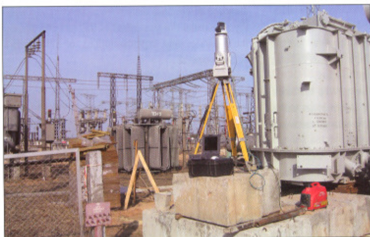
Figure 1: Laser Scanner RIEGL LMS-Z420i is on the high-voltage substation project.
